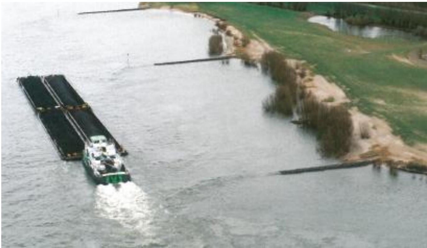
Effects of towboats with four loaded barges passing a groyne field in the River Waal
